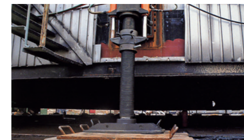
Replacing a tank side plate with the jacking method
