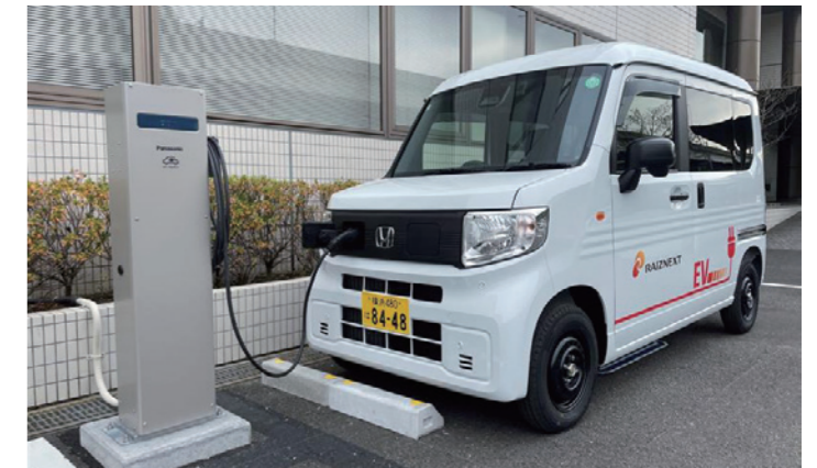
A company EV being charged
