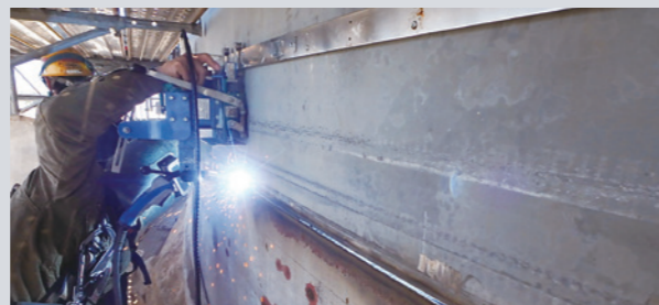
Welding tank side plates with an automatic welding machine
