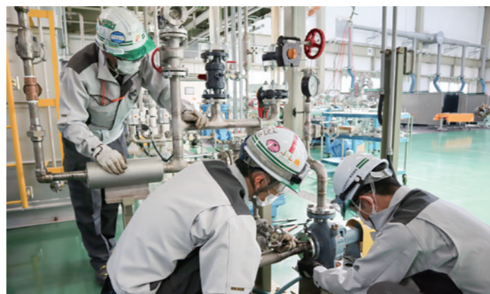
Training in a mock-up plant
